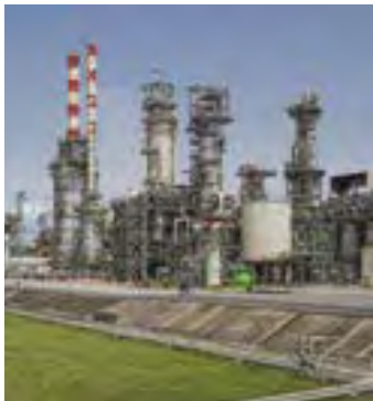
There is a brownfield plot available for the expansion of the Bonny Island liquefaction plant to eight trains
